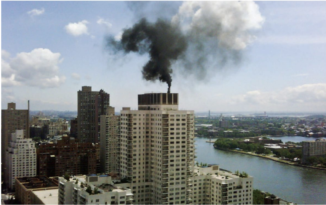
The black smoke commonly seen from New York City buildings using heavy heating oil (Source: Environmental Defense Fund)
