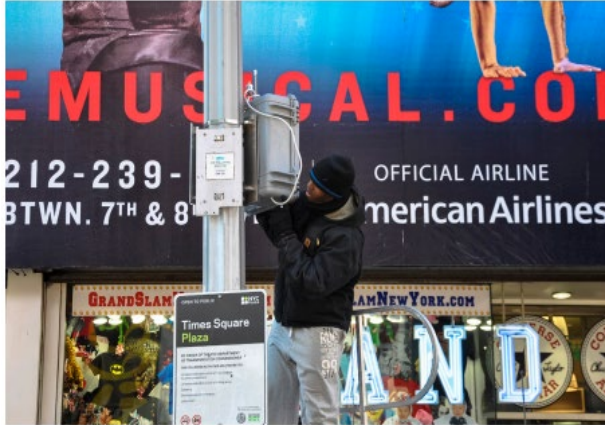
NYCCAS sensor on a lamp post in Times Square (Source: City of New York)
